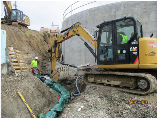
Clarifier Piping Installation
