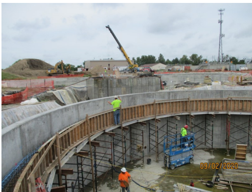
Clarifier Trough Construction- left
