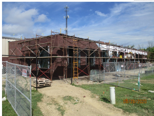
Office Masonry Exterior Installation
