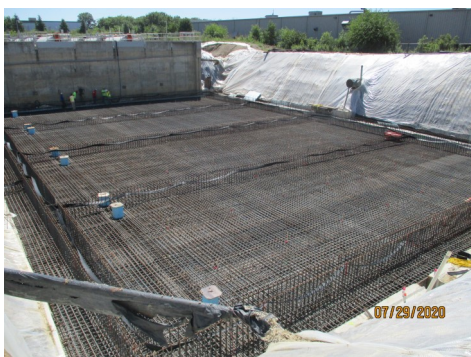
VLR slab rebar
