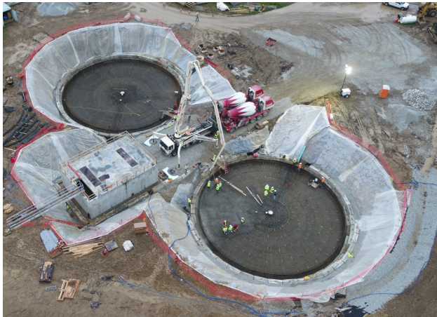
Clarifier Floor Slabs Being Poured
