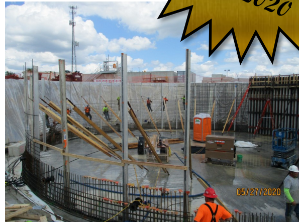
Clarifier Wall Rebar Installation
