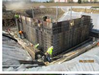
Left: Crews have been working hard on both the WRRF expansion project and the office remodel. These pictures show the assembling of forms and rebar for the RAS Pump Building foundation walls, an aerial view of the progress on April 29.
