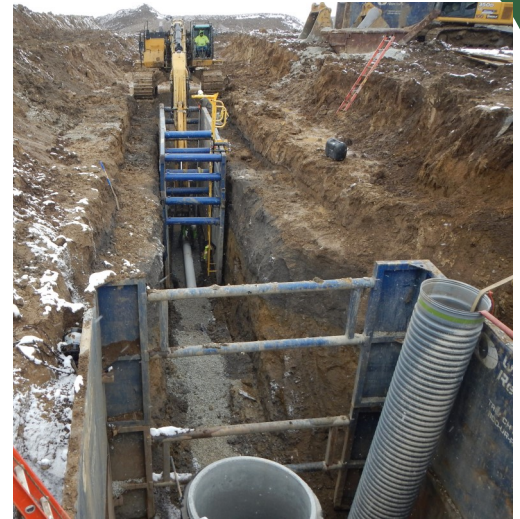
Deep Sewer Installation
