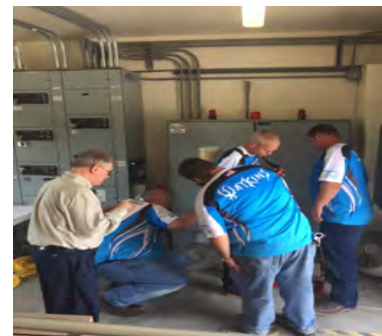
Completing in the Operations and Maintenance Event
