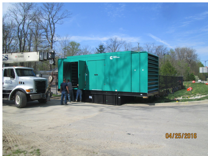
New 750 KW generator recently delivered to Lift Station 2.
