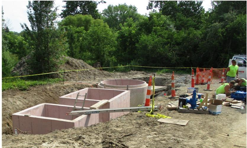
Lift Station 8 new wet well valve vault and meter vault installed.
