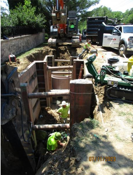
Lift Station 8 new ARV structure installed near 106th Street.
