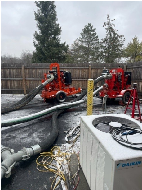
Bypass pumps at Lift Station 1
