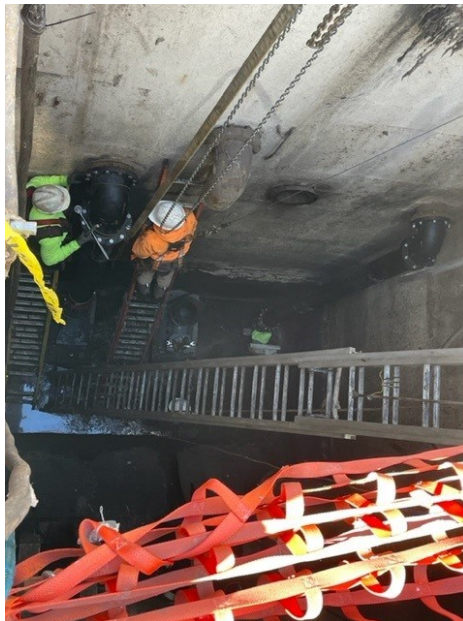
Installing Discharge Pipe Lift Station 1
