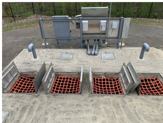
New Safety Nets Installed at Lift Station #10
