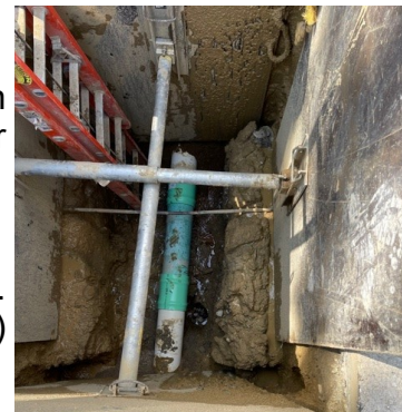
(Left) Damaged sewer main on Preston Drive from a contractor cross bore
