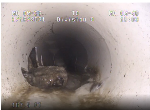
(Left) Damaged sewer main on Preston Drive from a contractor cross bore
