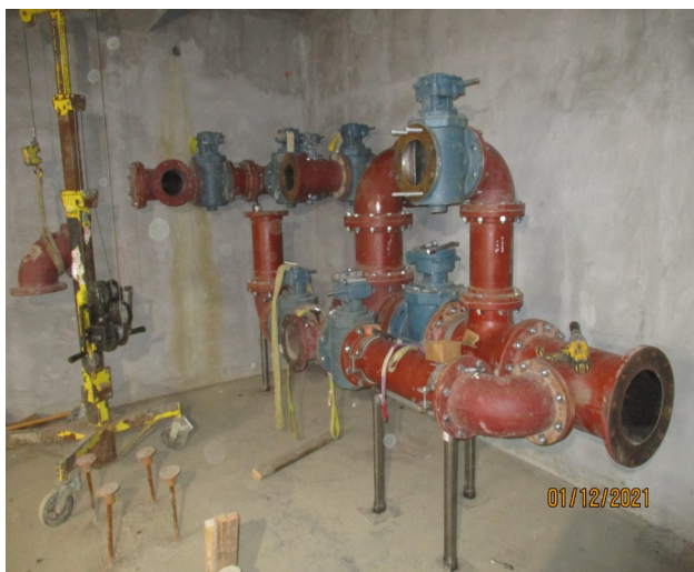
Process piping underway in the new RAS pump building
