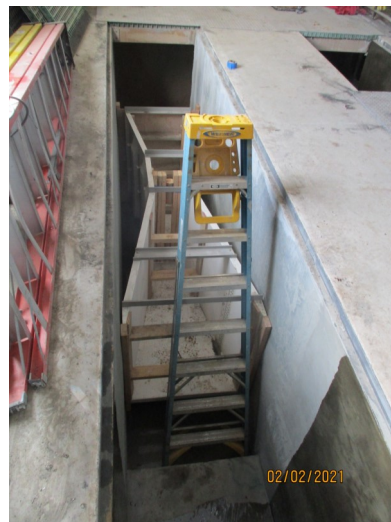
Channel lining and Parshall Flume installation in pretreatment
