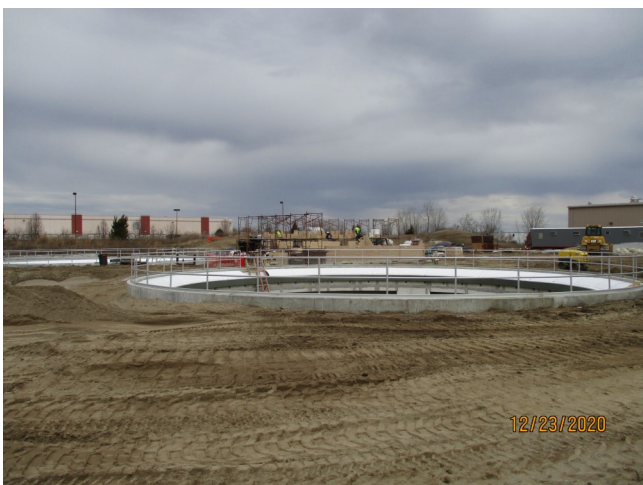
Backfilling new clarifiers
