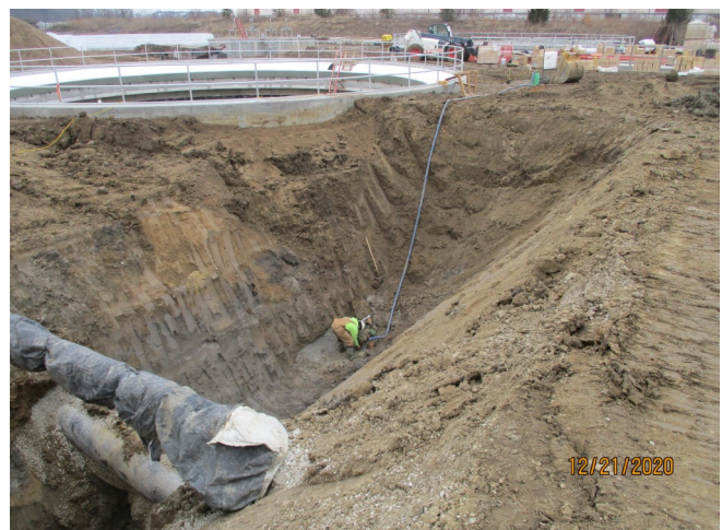
Plant-Yard piping installation
