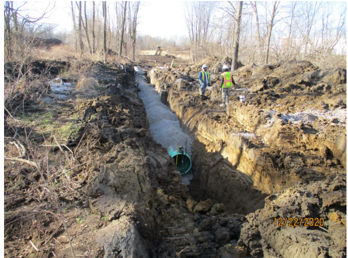
Outfall sewer installation
