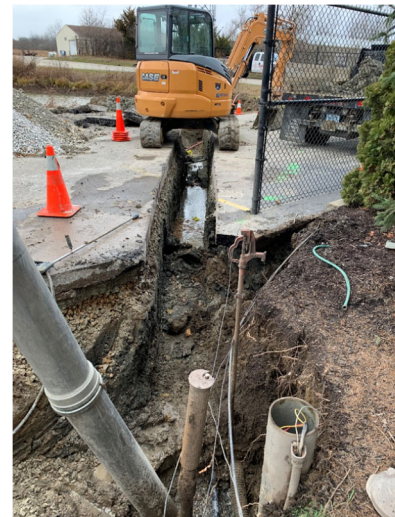
Well Line Replacement at the Plant
