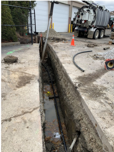
Well Line Replacement at the Plant
