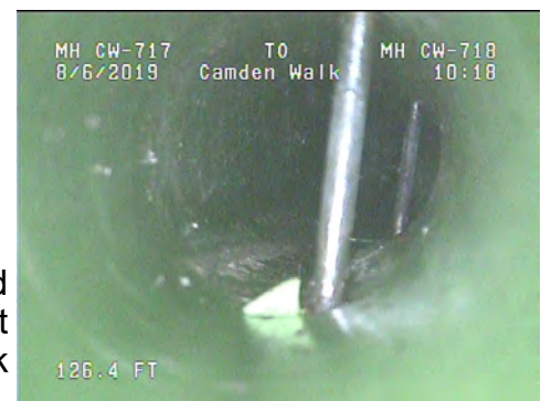
Grounding rods found in the sewer main at Camden Walk
