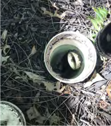
Photo to the left: Illegal connection of a downspout into the cleanout.
