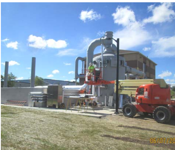
WWTP Odor Control Project: Working on pipe and duct insulation
