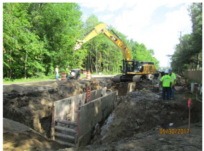
Springmill Parallel Interceptor Project: Gravity sewer installation
