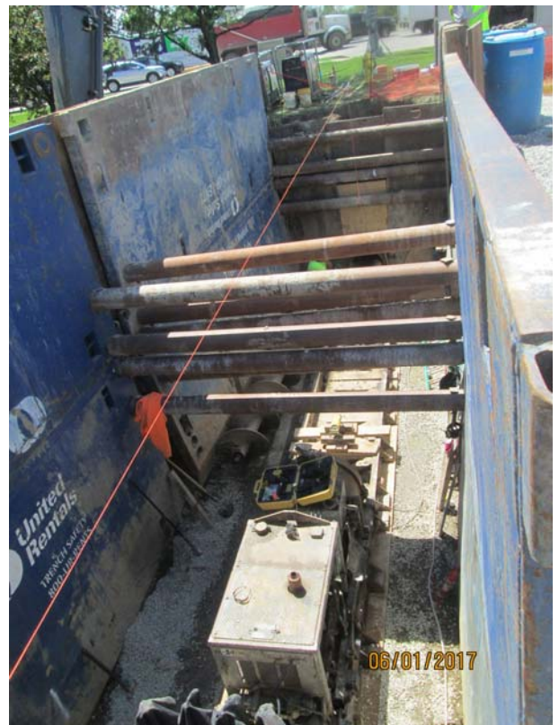
106th Street Parallel Force Main Project: Jack and bore installation underway across Michigan Road
