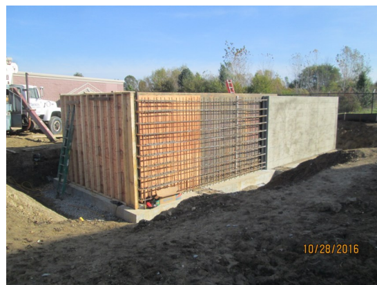
Crews constructing the biofilter tanks for the WWTP Odor Control Upgrades project.
