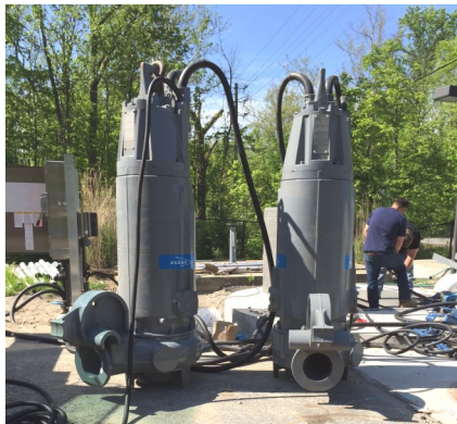
New 335 Hp Pumps that will send flow to Michigan Road WWTP from Lift Station 2
