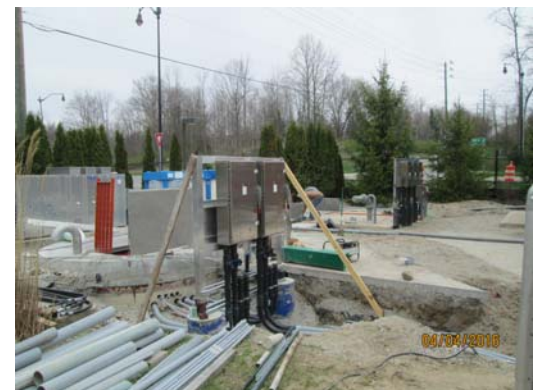
Disconnect Stands at both Lift Station 2 wet wells
