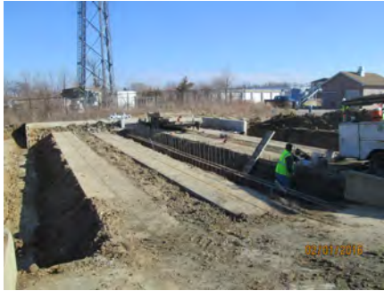
Drying Bed wall reconstruction underway at the Michigan Road WWTP
