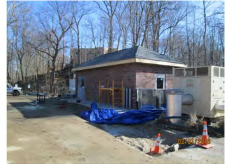
Lift Station 2 Upgrades project: Completed walls and roof for the new electrical building
