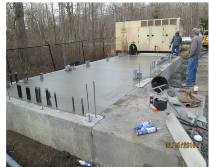
Lift Station 2 Upgrades Project: Foundation walls and floor slab concrete poured; ready for block walls construction at the new electrical building.
