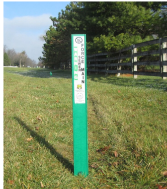
Above-ground warning marker installed over a force main along Clay Center Road.
