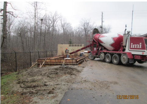
Crews constructing foundation walls for the new electrical building at Lift Station 2 (Springmill/106th)
