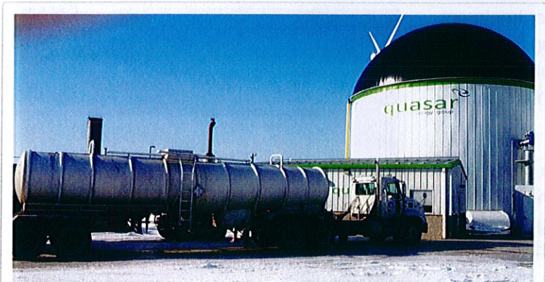
This Quasar Energy Group (Cleveland) facility uses anaerobic digestion to treat the Village of Swanton's (Ohio) biosolids and produce methane. Photo courtesy of the Quasar Energy Group.
