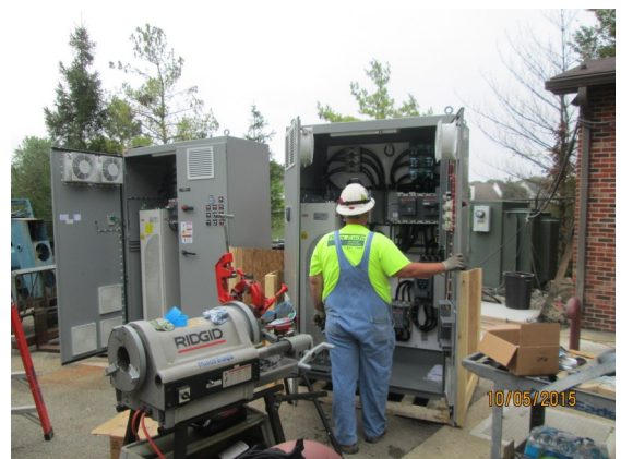
Preparing the new large VFD's for installation at Lift Station 1
