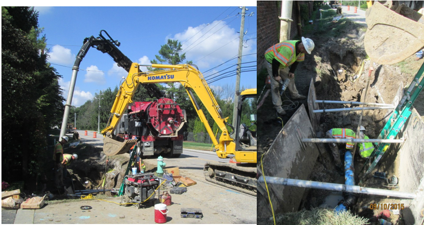
Force main relocation underway along 106th Street at Laurelwood. This line was in the way of retaining walls needed for Carmel's future multi-use path.
