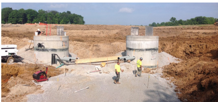
Preparing subgrade for the valve and meter vaults at the Northeast Regional Lift Station. The two completed wet wells are in the background.
