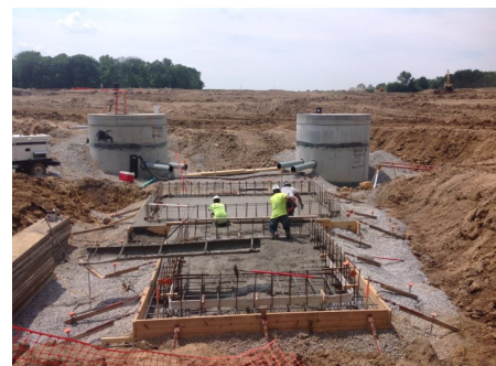
Pouring the concrete floor slab for the valve and meter vaults at the Northeast Regional Lift Station.
