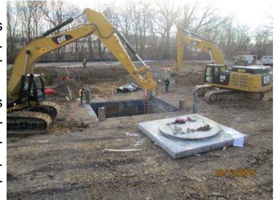
Crews are preparing to set the 38,000 pound precast concrete base (foreground) for the wet well.
