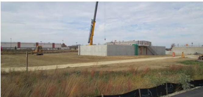
Final grading is underway around the new digesters at the plant. The crane is lifting the last pieces of equipment into the tanks for installation.
