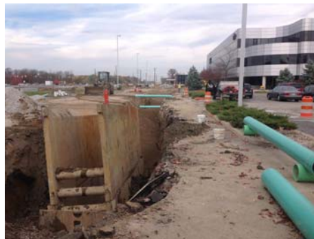
Sewer relocation work continues near the southeast corner of US 31 and 106th Street
