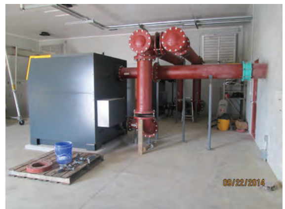
Installation of two new 175 Hp blowers and air piping that will service new digesters at the plant. The blowers are about 7 feet tall.
