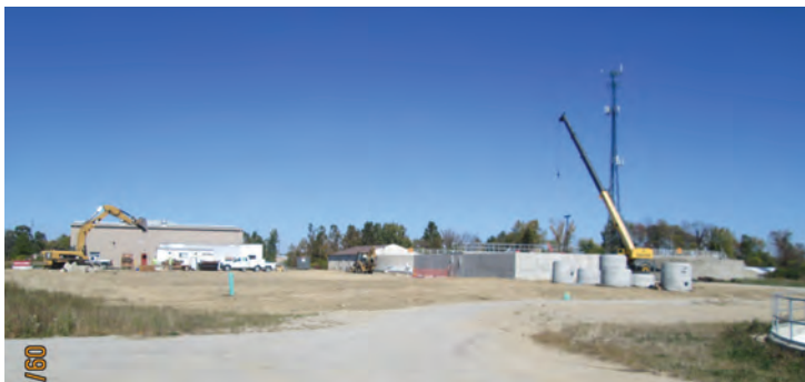
Final grading underway west of the new digesters after over 3,000 cubic yards of soil stockpiled on site was hauled away. The existing Biosolids Building is on the left and the new digesters are on the right.
