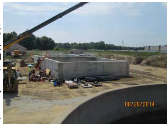
Piping and equipment installation underway at the new digesters (Biosolids Improvements project).
