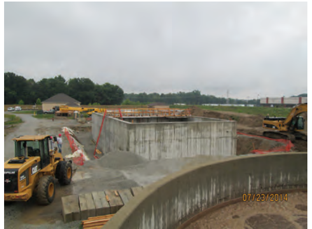
Concrete work on the new digester is nearly complete (view is looking south from the bridge over Digester 3.)
