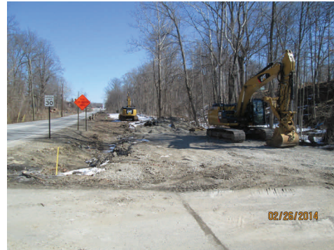
Looking east along 106th St. from LS #2—trees and shrubs cleared from the gravity sewer and forcemain relocation routes
