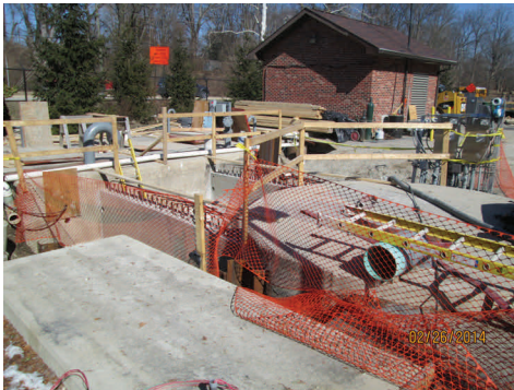
Construction of the new splitter at LS #2
