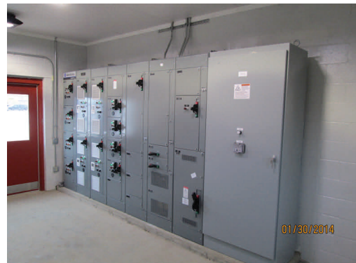
Electrical equipment inside the new VLR Control Building
