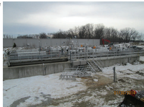
Four VLRs and anaerobic zones operational
